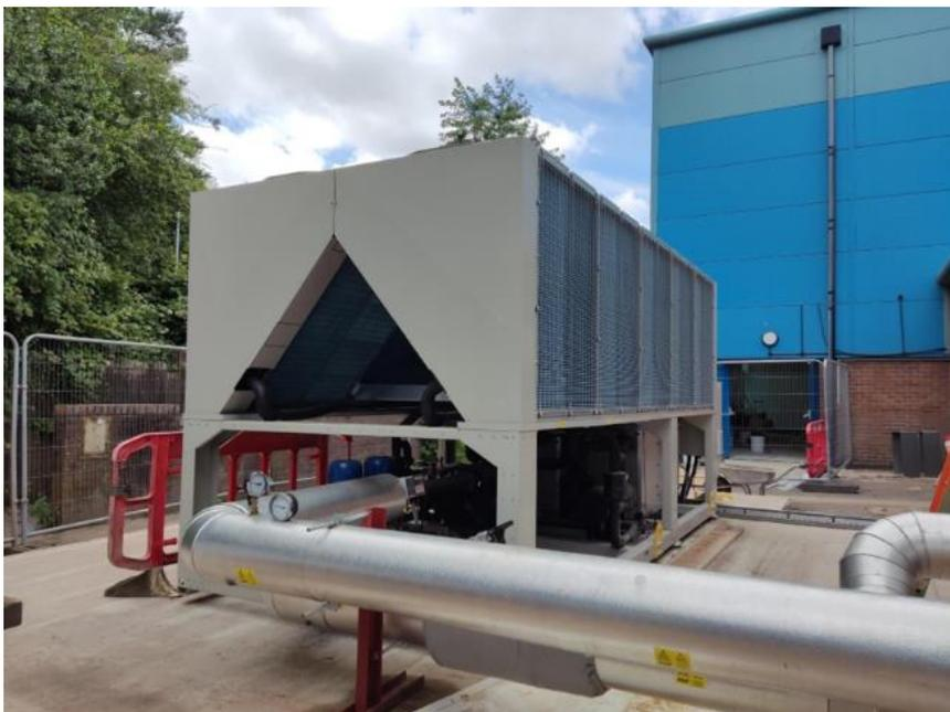
*Figure 4 Recently installed Air Source Heat Pump at Oakengates Leisure Centre.*
